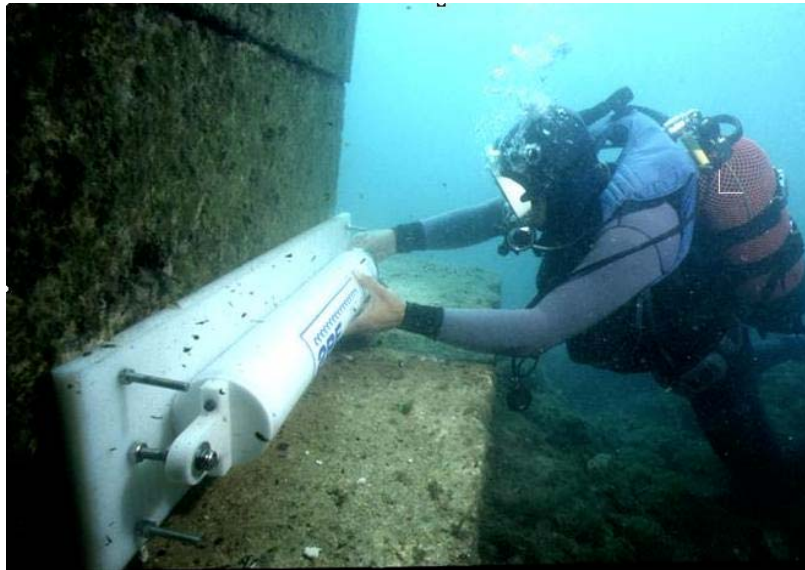
Figure 6 The installation of a SBE tide gauge requires the hiring of divers. In the pilot station, the sensor was placed inside a protective PVC tube.
