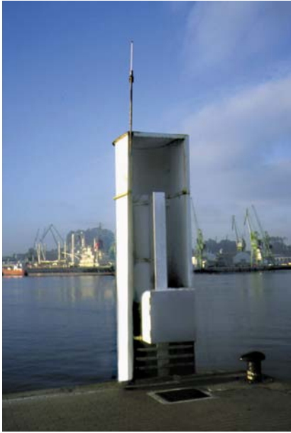
Figure 8 SRD station in the harbour of Vilagarcía de Arousa
