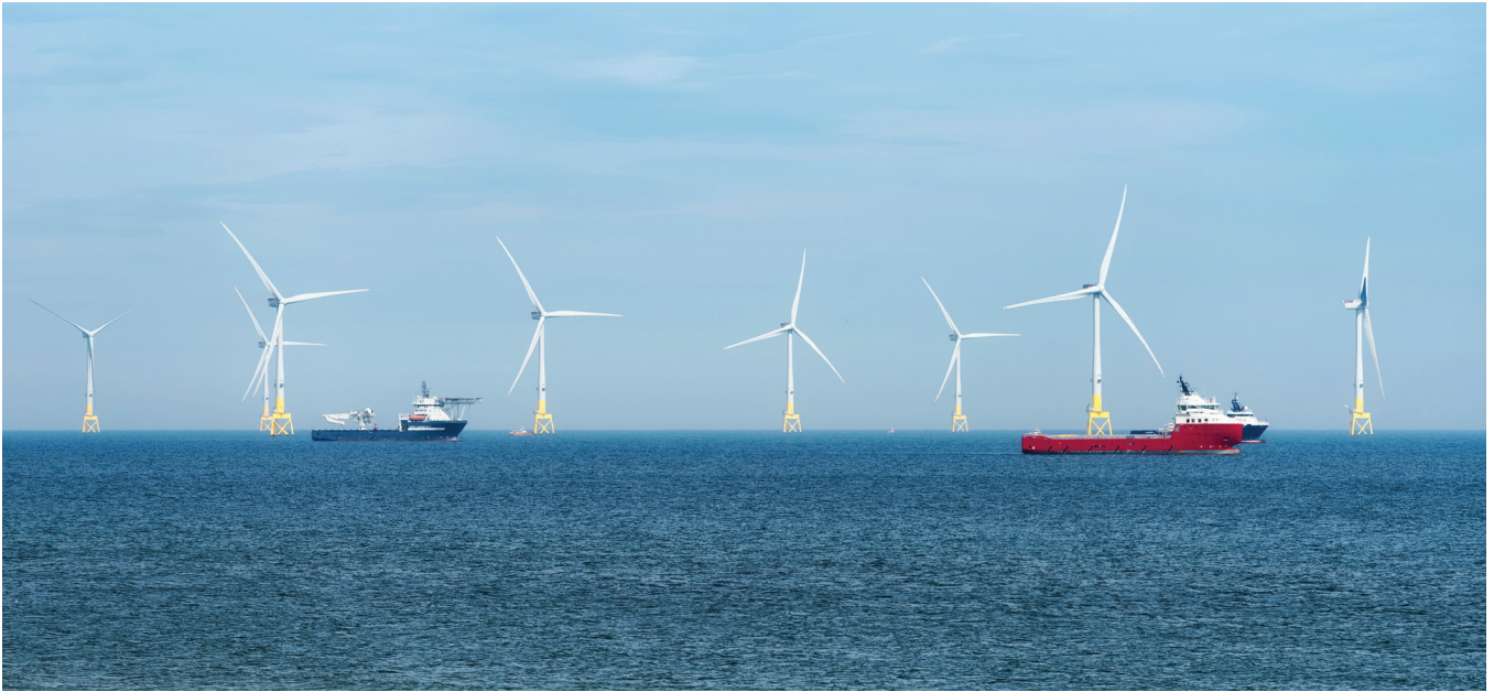
Mitigate challenges. Whether it is crane operations or cable laying, mobilising personnel at the right moment relies on the accessibility to immediate and reliable sea state data
